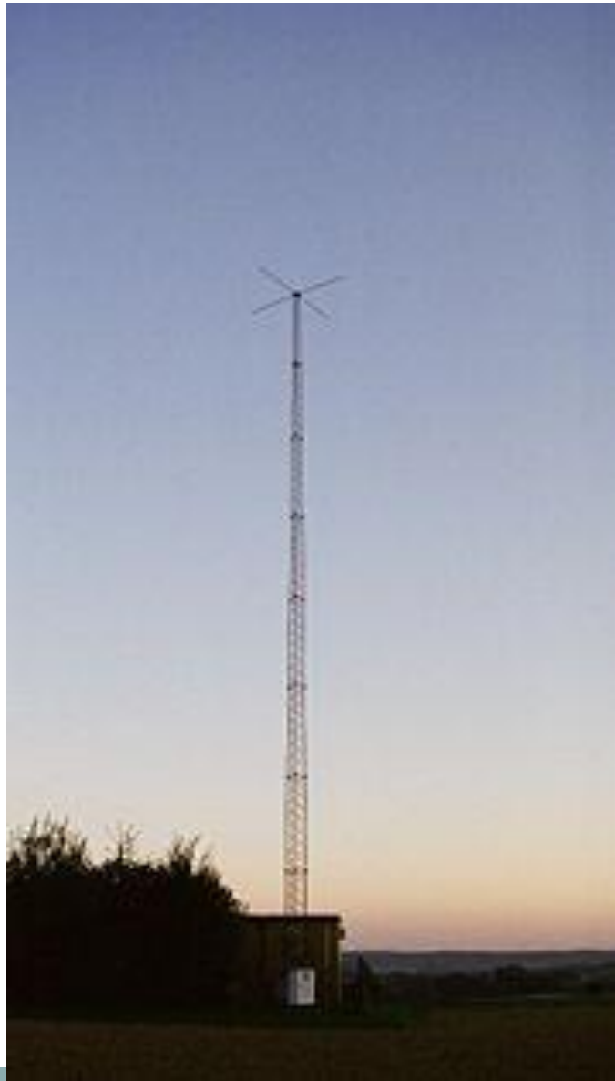
Non Directional Beacon
